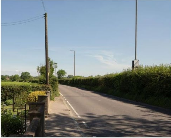
Existing North Road, north of South Ockendon
